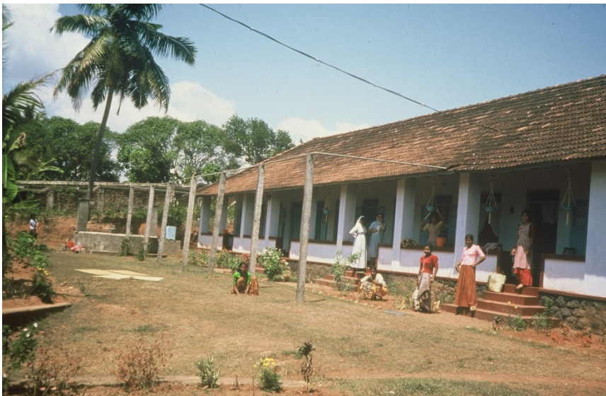
Figure 58: The first house in Villoomni
