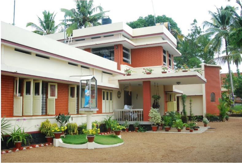
Figure 59: The Regional House in Villoonni
