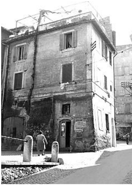
Novitiate House in Tivoli 1 st floor, Piazza Colonna 1899-1904
